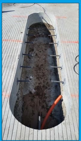
Directional drill machine pulling in new HDPE conduit & 1/0 counterpoise under the Runway
