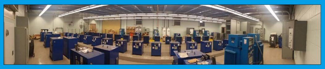
The CCRs are laid out so the taxiway CCRs are in the middle of the vault on the raised step and runway CCRs are on the perimeter of vault room.
