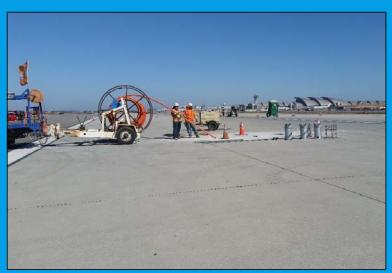
Installation of HDPE conduit by horizontal directional drilling under the runway
