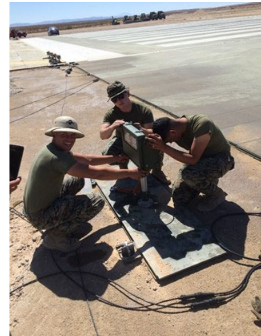
MWSS-374 Marines installing REIL
