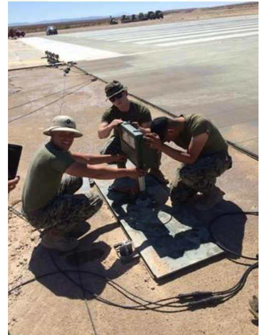
MWSS-374 Marines installing REIL
